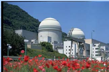
Takahama Power Station
