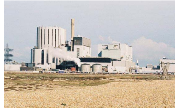
Dungeness B (UK) uses advanced gas-cooled reactor
