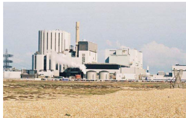
Dungeness B (UK) uses advanced gas-cooled reactor
