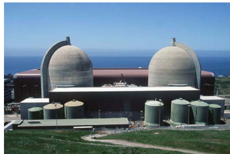
Diablo Canyon(USA) 4-loop pressurized water reactor
