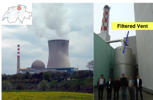
Fig. 17 FCVS in Leibstadt NPP (BWR), Switzerland [6] .
