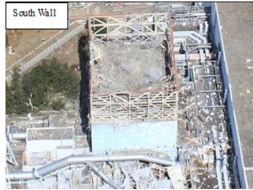
Fig.9 Appearance of Unit 1 R/B after explosion.
