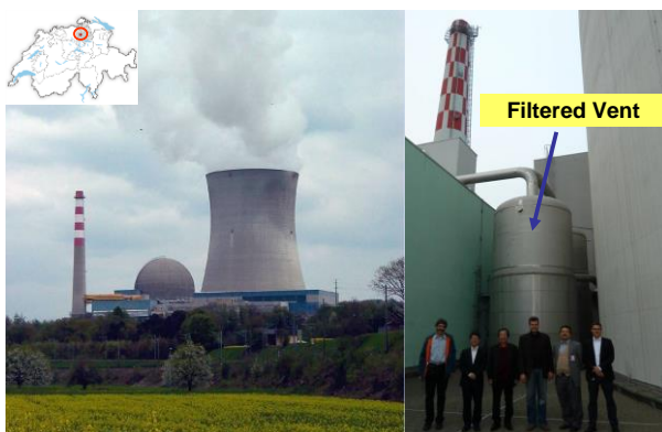
Fig. 17 FCVS in Leibstadt NPP (BWR), Switzerland [6].
