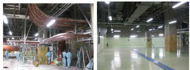
Before dismantling work
