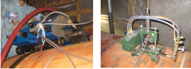
Fig.5 Cutting work of feed water heaters.
