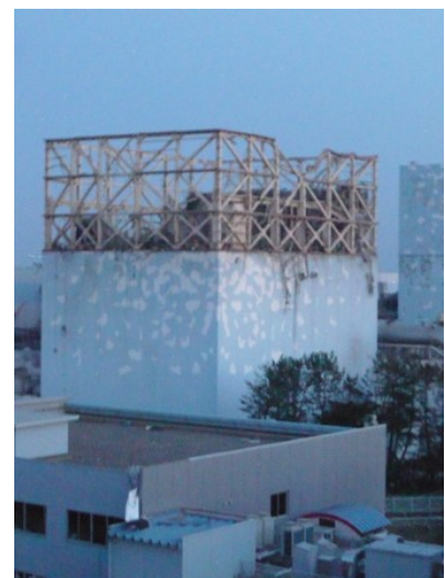
Fig.11 Photo showing exterior view of reactor building of the Fukushima Daiichi NPS (Unit 1) after hydrogen explosion. Reference: TEPCO Release [online] http://www.tepco.co.jp/tepconews/pressroom/110311/
